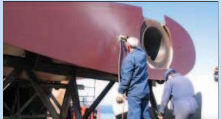
Corrosion inhibitor is blown into the rudder through openings.
