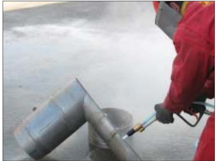
Figure 10. Surface preparation with wet blasting process
