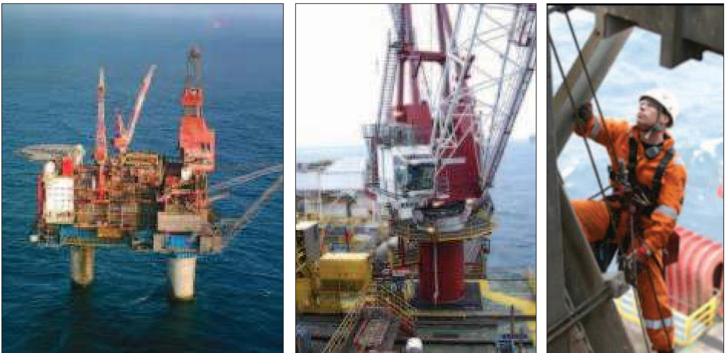
Figure 13. Drilling platform “Gullfaks B”
