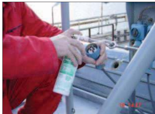
Image 18.b Applying VpCI® 238 for protection of electric contacts
