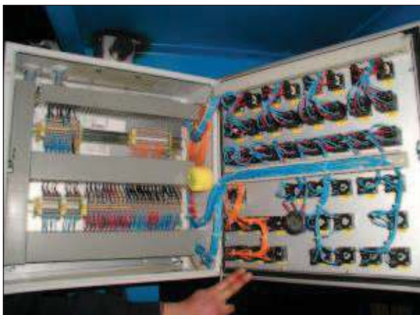
Image 18.a Applying VpCI® Emitter in electric panel
